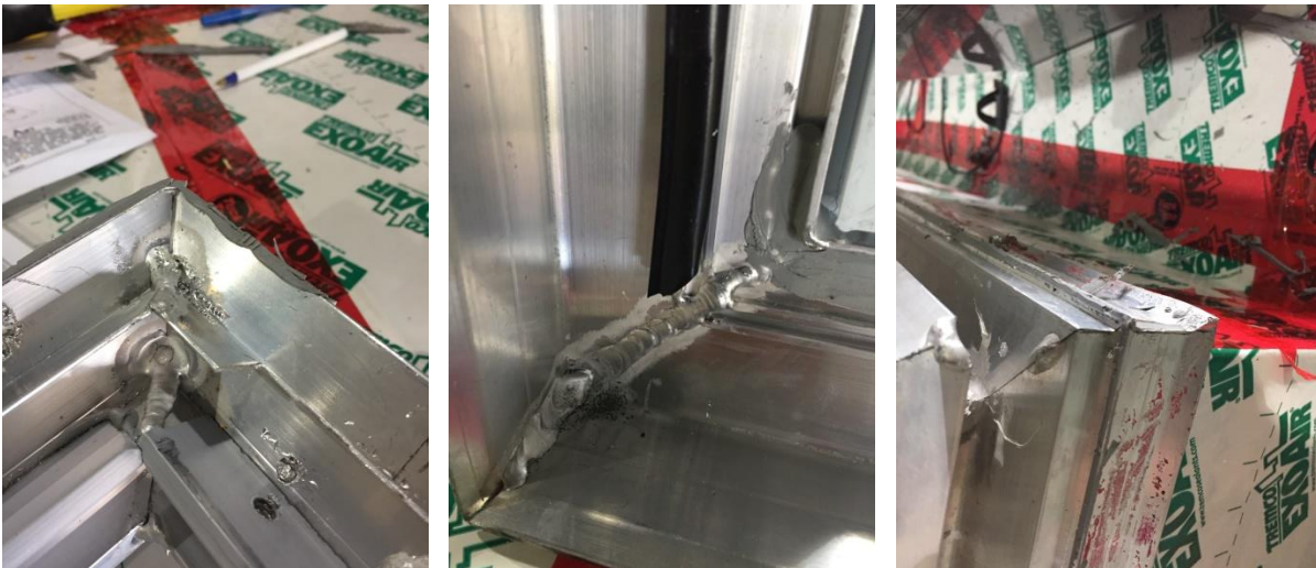
Curb Frame Corner Weld Details
