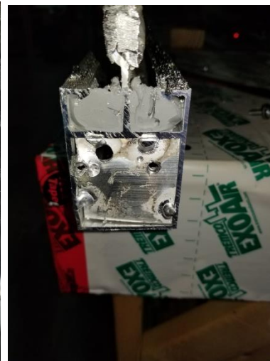
Photo 8- Angle bracket at ridge end of intermediate rafters.
