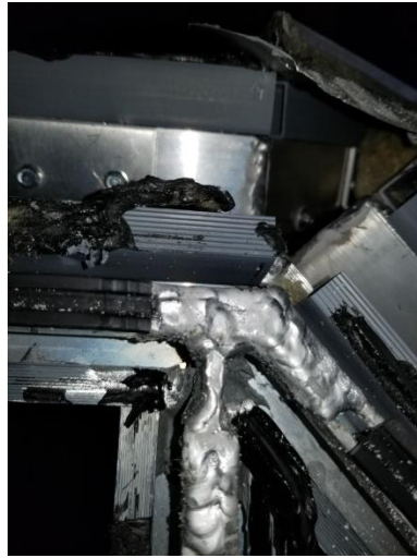
Photos 11 and 12- The intersecting end rafters were welded together across the pressure plate screw-port portion of the extrusion and along the outside edge of the corner joint. The outer glazing legs of the intersecting rafters were also welded together along the apex.
