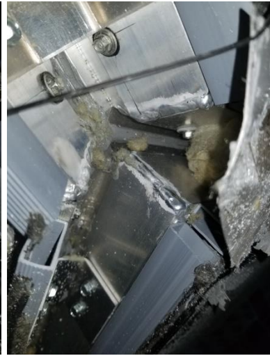
Photos 11 and 12- The intersecting end rafters were welded together across the pressure plate screw-port portion of the extrusion and along the outside edge of the corner joint. The outer glazing legs of the intersecting rafters were also welded together along the apex.
