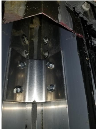
Photo 7- Ridge rafter to intermediate rafter fasteners. and 'V'-shaped ridge rafter connection plate.
