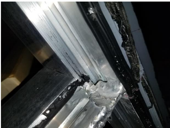
Photo 7- Ridge rafter to intermediate rafter fasteners. and 'V'-shaped ridge rafter connection plate.
