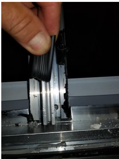
Photo 6- Curb frame to rafter fasteners- two per end of rafter.
