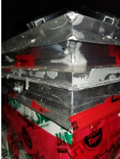
Photo 3- Curb frame corner weld details.
