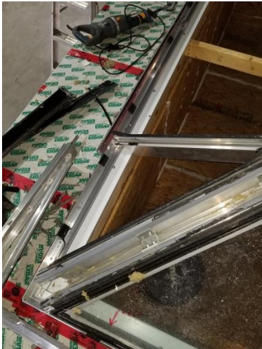
Photos 13 and 14- Two 'V'-shaped 3.2 mm thick aluminum connector plates secured the adjacent rafters together at each corner. At the curb end of each corner, the adjacent rafters were joined using a brake-formed 'V'-shaped connector plate formed from 27 ga aluminum sheet.
