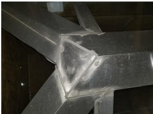
Photos 13 and 14- Two 'V'-shaped 3.2 mm thick aluminum connector plates secured the adjacent rafters together at each corner. At the curb end of each corner, the adjacent rafters were joined using a brake-formed 'V'-shaped connector plate formed from 27 ga aluminum sheet.
