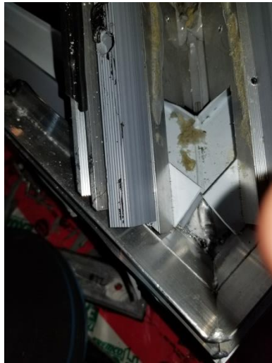
Photo 4- Curb frame corner weld details.
