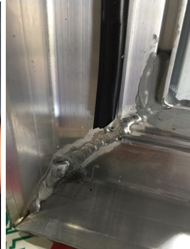
Photo 5- Curb frame corner weld details.
