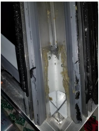
Photos 13 and 14- Two 'V'-shaped 3.2 mm thick aluminum connector plates secured the adjacent rafters together at each corner. At the curb end of each corner, the adjacent rafters were joined using a brake-formed 'V'-shaped connector plate formed from 27 ga aluminum sheet.
